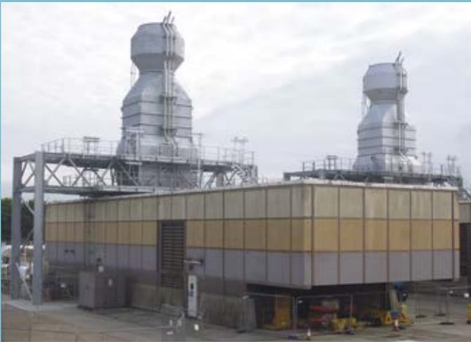
New exhaust stack and catalyst abatement system at Aylesbury compressor station.
