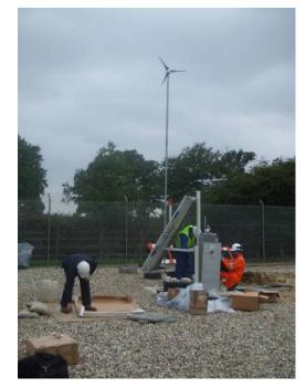
Fig 2 – Hydrophone installation at one of the sites
