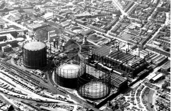
Figure 19. Views and a sketch of Windsor Street gasworks. Top – Panorama across the works 1928 Middle – Sketch of the gasworks from the entrance c1928; Bottom Left – an aerial view of the gasworks c1950 Bottom Right – A view of the gasworks c1940 showing the purifiers, new coke plant and cooling tower in the foreground. Source: National Grid Gas Archive.
