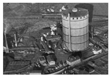
Figure 23a. Aerial view of the gasworks showing the MAN waterless gasholders. Source: National Grid Gas Archive.
