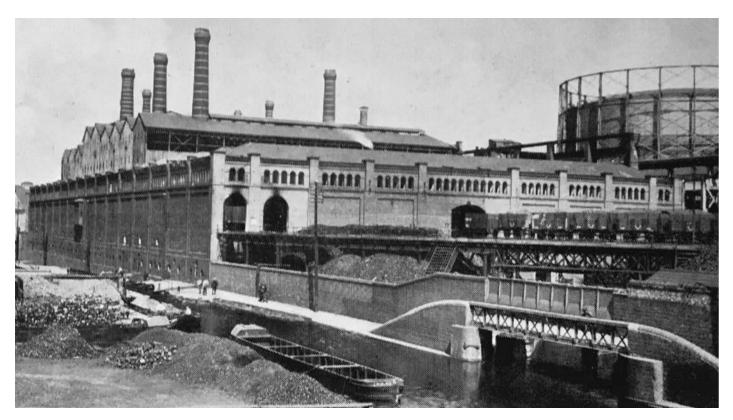
Figure 17. The canal with retort house behind. The taller vertical retorts can be seen to the back of the retort house with the tall chimneys. Source: IGEM Archive.
