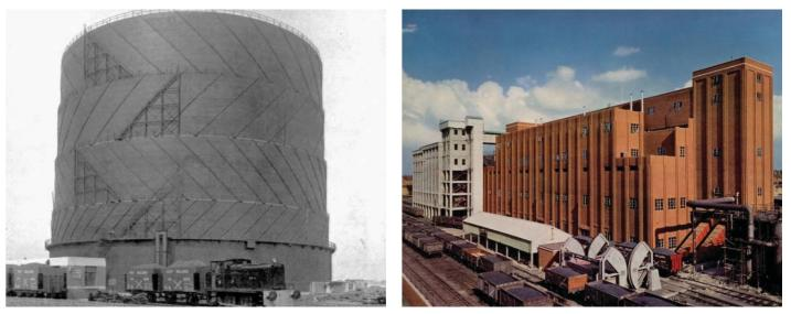
Figure 23b. Views and a plan of Swan Village Gasworks. Top - a plan of the old and new gasworks c1953 Middle - Panorama across the old gasworks c1928. Bottom Left - the spiral guided gasholder. Bottom Right - a view of the new vertical retort house built for the West Midlands Gas Board, with the railway in front. Source: National Grid Gas Archive.
