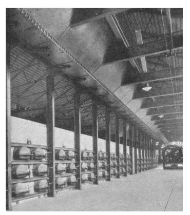
Figure 26b. A view of the retorts and charging machine at Adderley Street Gasworks c1928. Source: National Grid Gas Archive.
