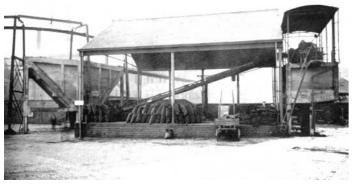
Figure 26c. The coke bagging plant at Adderley Street Gasworks c1928. Source: National Grid Gas Archive.
