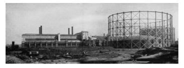
Figure 43. Nechells gasworks c1928, showing the No.1 retort House (left) and the No.6 and No.5 gasholders (right). Source: National Grid Gas Archive.
