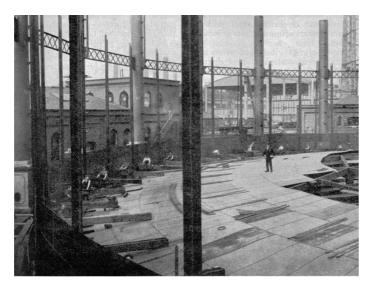
Figure 18. Reconstruction of Gasholder No.12, during the lowering of the 2nd lift. Source: National Grid Gas Archive.
