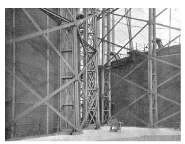
Figure 12. The point at which the twin gasholders meet at the Windsor Street Gasworks c1902. Source: National Grid Gas Archive.
