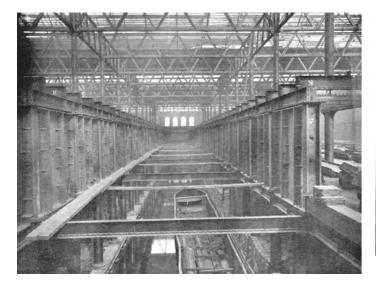
Figure 13. The interior of the retort house during construction, showing the integrated connection between the canal basin and retort house, c1902, Source: National Grid Gas Archive.
