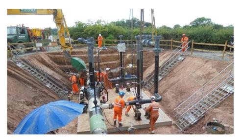
Figure 17: Installation of Dymock pipework arrangement
