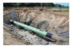
Figure 20: Excavated Deerhurst West site with previous block valve, and new pipethrough
