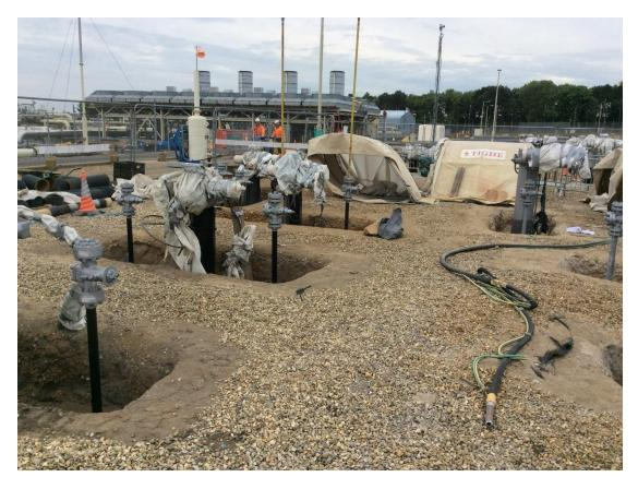
Figure 9: Wind/waterline paint inspection in progress in Perenco manifold area
