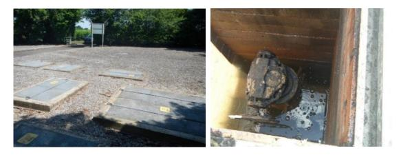
Figure 16: Dymock AGI with deep pits exhibiting gas leaks
