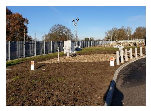
Figure 26: Completed King's Lynn valve works including new test posts
