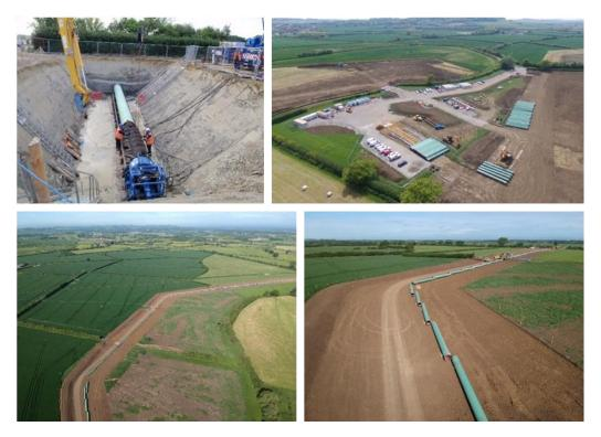
Figure 37: TX01 Diagrams. (a) Auger Bore Set up at road crossing; (b) Site Establishment; (c) and (d) – Ariel view of pipeline routing following top soil strip and pipe string activities
