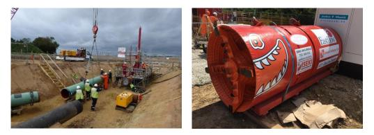
Figure 39: Diversion works completed via micro-tunnel
