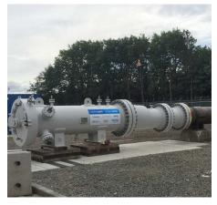
GRAID launch vessel connected to the NTS.
