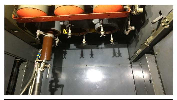
TO REMOVE CARRY OUT ABOVE SEQUENCE IN REVERSE. ENSURE TEST BUSHING IS REMOVED FIRST. PRIOR TO REMOVAL OF EARTH CLAMP. FURTHER INFORMATION ON TEST BUSHINGS CAN BE FOUND ON AEI DRAWING A2323251 (TYPE VSLP9-15 ARRANGEMENT OF MAIN SPOUT TEST STICKS).
