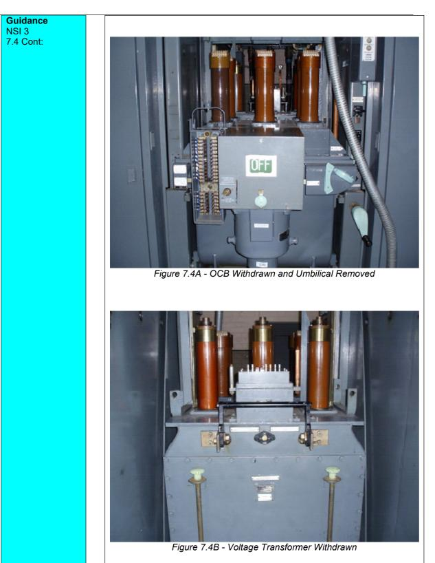
Note: the primary (rear) and secondary (front) connections are automatically broken by withdrawing the  $\mathsf{VT}$
