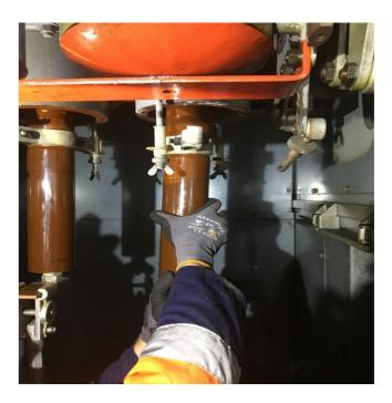
APPLY TEST BUSHING SECURING BOLTS (2 OFF ADJACENT TO EACH OTHER) TO EACH SPOUT FLANGE I.E. 6 OFF SECURING BOLTS. APPLY ONE TEST BUSHING AT A TIME, OFF SET SLIGHTLY FROM MID-POINT CLAMP PUSH UPWARDS & TWIST TO ENGAGE CLAMP WITH SECURING BOLTS. SECURE TEST BUSHING IN PLACE TIGHTENING UP THE TWO BRASS CLIPS/NUTS/WING NUTS.
