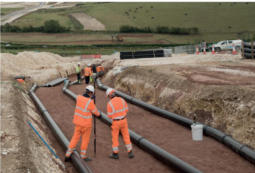
Cables will be installed 1.5 metres underground, as seen in the above image.
