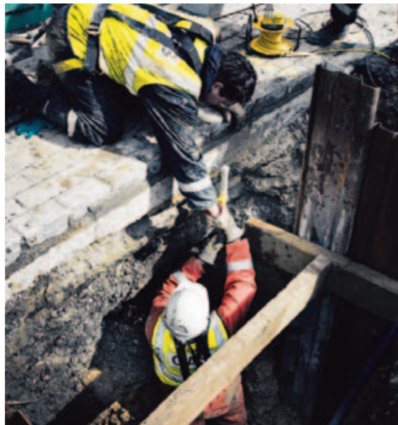
▣ Repairing a gas escape in the highway.
