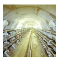
Internal view of high voltage underground cable tunnel.
