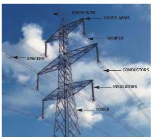
The components of overhead power lines.
