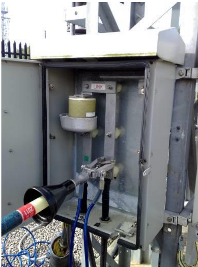
Figure 6.1C - Temporary Earth Bond
