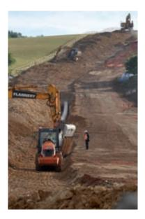
**WORK IN PROGRESS:** National Grid is currently working on a new 48-inch gas pipeline from Wormington to Sapperton, near the Cotswolds stables
