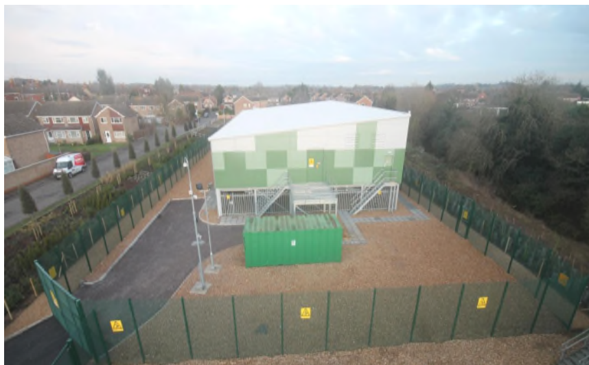
Image 1 (courtesy of UKPN): Smarter Network Storage (SNS) at Leighton Buzzard (6MW, 10MWh, Li-NMC).
