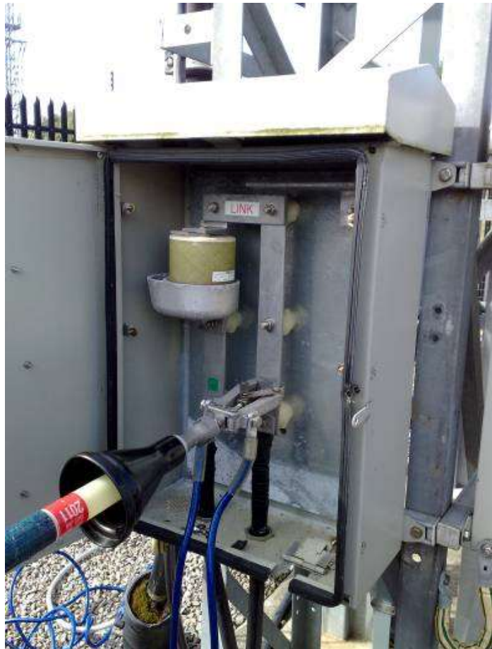
Figure 6.1C - Temporary Earth Bond
