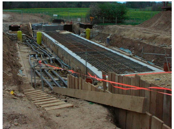
Stop joint with adjacent fluid tanks under construction
