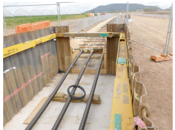
Direct buried cable installation in a rural area
