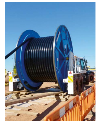
Cable drum offloading cable on site
