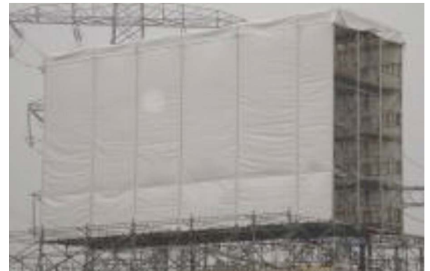
A sealing end compound under construction
