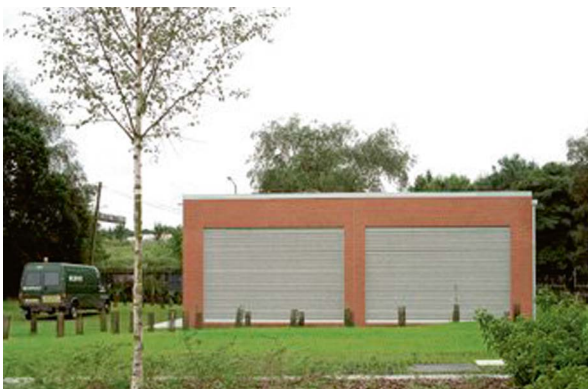
Tunnel head house building
