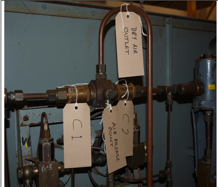
Figure 5.3A – Example of physically identifying the point(s) at which the Equipment is to be vented using temporary labels
