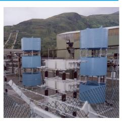
Air Core Reactors (blue), image courtesy of Enspec Power
