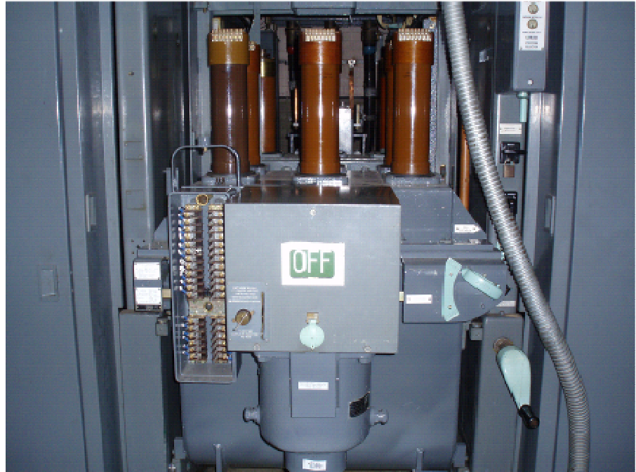
Figure 7.4A - OCB Withdrawn and Umbilical Removed
