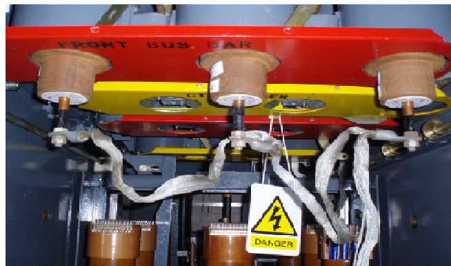
Figure 5.4A - Metalclad Switchgear Moveable Earths
