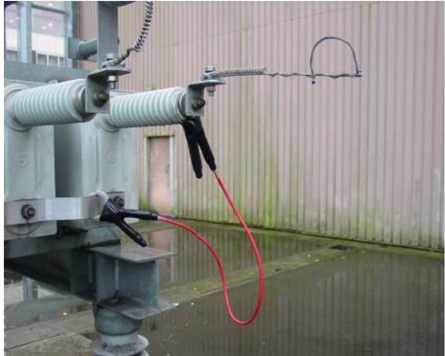
Figure 6.3A – Applying the Clip-on Short Circuited Lead
