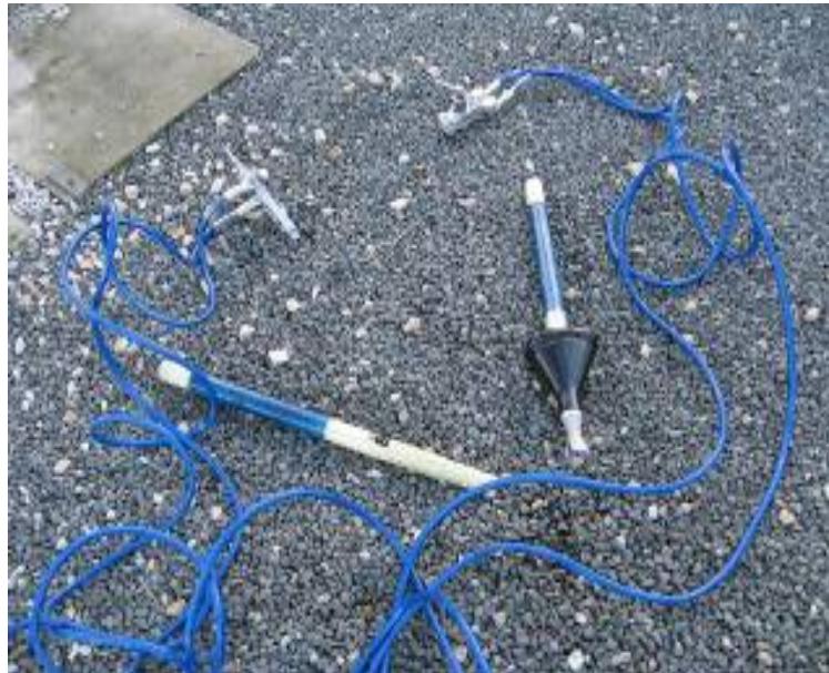
Figure 6.2A - Temporary Earth Bond and Pole
