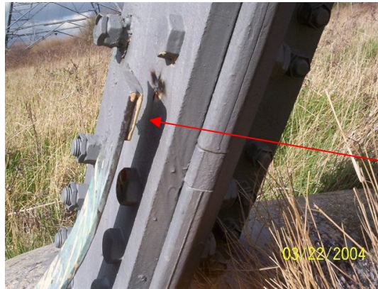
Figure 8.4 - Example Defective Earth Tape Connection
