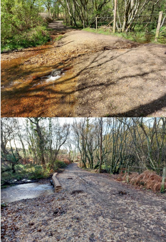
Figure 4.10 New Forest National Park: New Forest Access and Landscape Enhancement - culvert repairs and path re-instatement.
