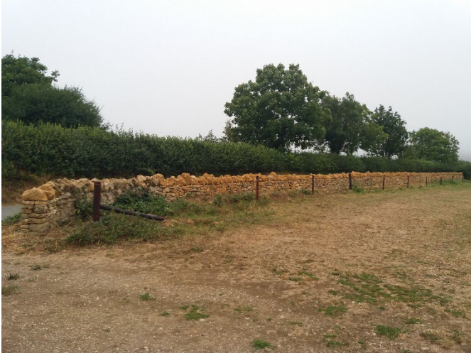
Figure 4.11 Dorset National Landscape: Reconnecting the Ridgeway - stone wall restoration.
