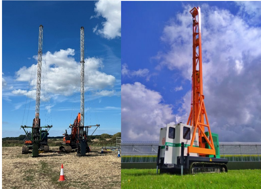
Equipment for ground investigation works
