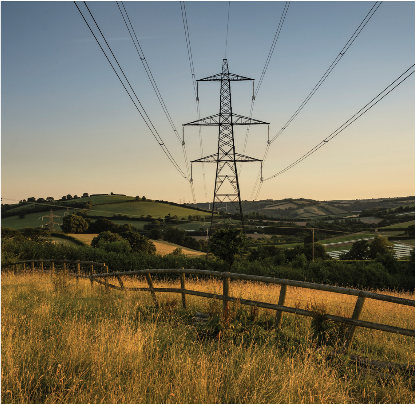
Figure 8 – Example of 400 kV overhead line and traditional steel lattice pylon – for illustrative purposes only
