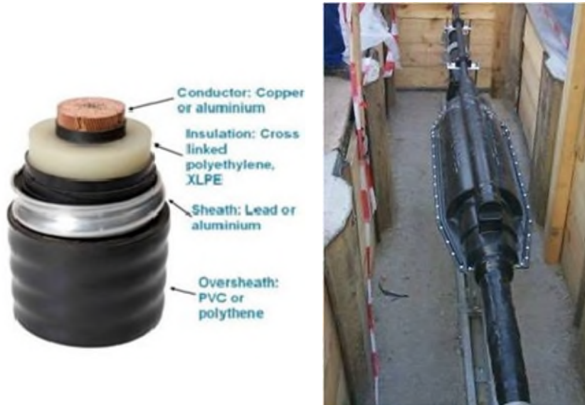
Figure C.4: Cable Cross-Section and Joint
