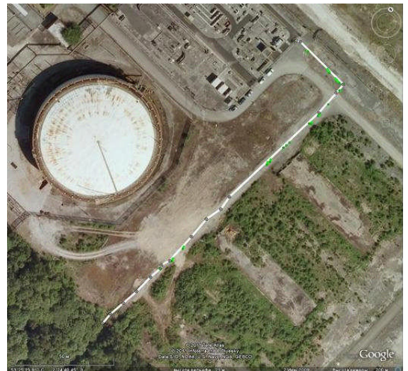
Warburton Pipeline showing locations of green anomalies identified during inspection
