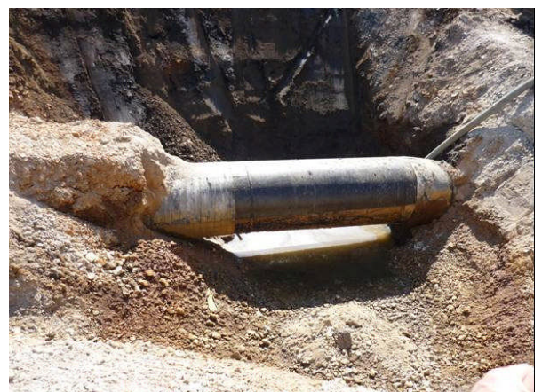
Section of excavated pipeline
