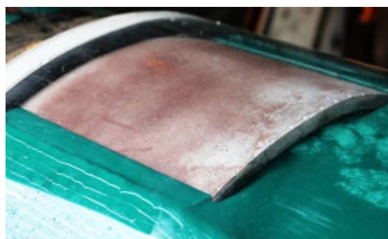
Polymer trial, three weeks after installation of the replacement material
