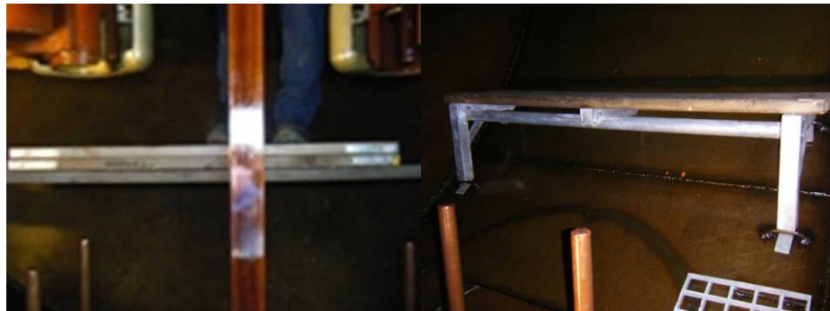
Temporary Work Bench showing Flooring Temporary Access Platform
