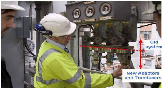
Single fitting adaptor for top-ups with transducer
