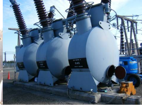
JW 420 Bulk Oil CB Tanks
