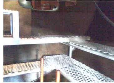
Temporary Access Platform
