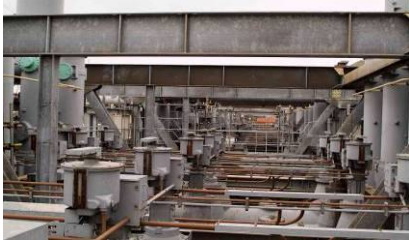
Site is large and difficult to retro-fit
