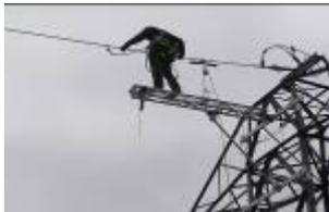
**Earthwire Platform** – this platform is being developed to provide a suitable access/egress platform whilst carrying out maintenance on earthwires. The initial prototype has been trialled, identifying a change to the specification and design parameters. The second prototype has been manufactured and tested. Field trials are to be completed to ascertain the suitability of the current design and any required design changes.
