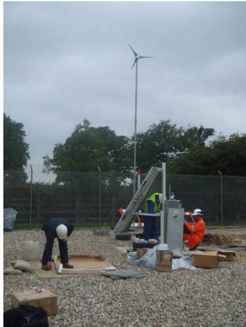
Fig 2 – Hydrophone installation at one of the sites
