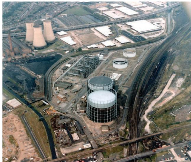
**Figure 79. The Washwood Heath site in the early 1970s showing the two gasholders and reforming plant. Source: National Grid Gas Archive.**
