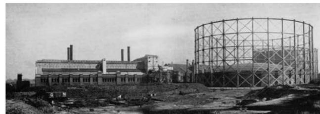
**Figure 43. Nechells gasworks c1928, showing the No.1 retort House (left) and the No.6 and No.5 gasholders (right). Source: National Grid Gas Archive.**
