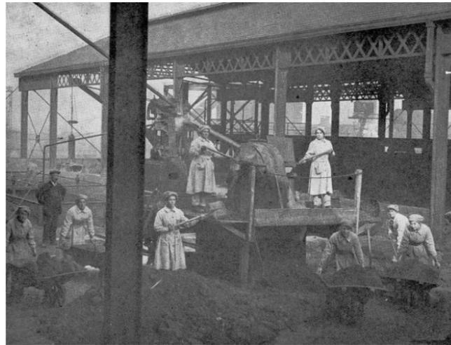
Figure 56. Female gas workers working on the Oxide Crusher at Nechells Gasworks, Birmingham, 1918, during World War I. Source: National Grid Gas Archive.
