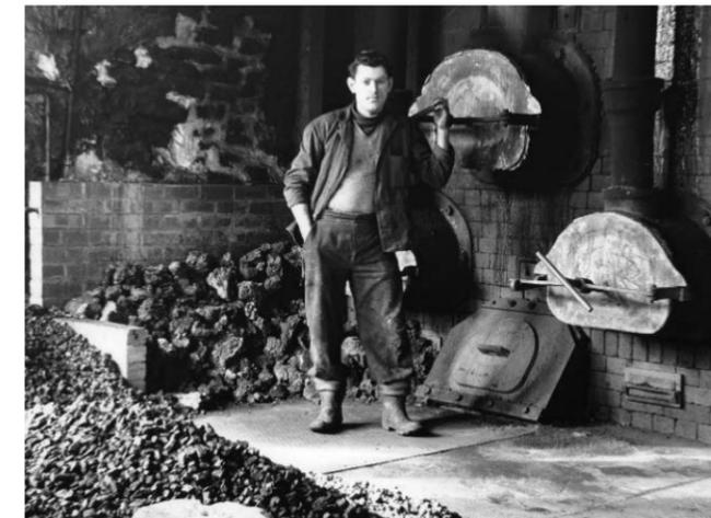
**Figure 81. The stoker and horizontal retorts at the small, former gasworks at Robin Hood's Bay, Yorkshire. Source: IGEM Archive.**
