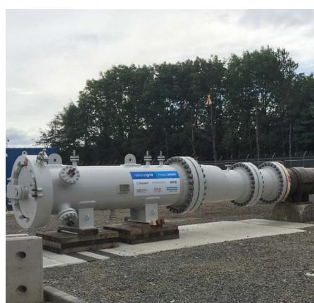
GRAID launch vessel connected to the NTS.
