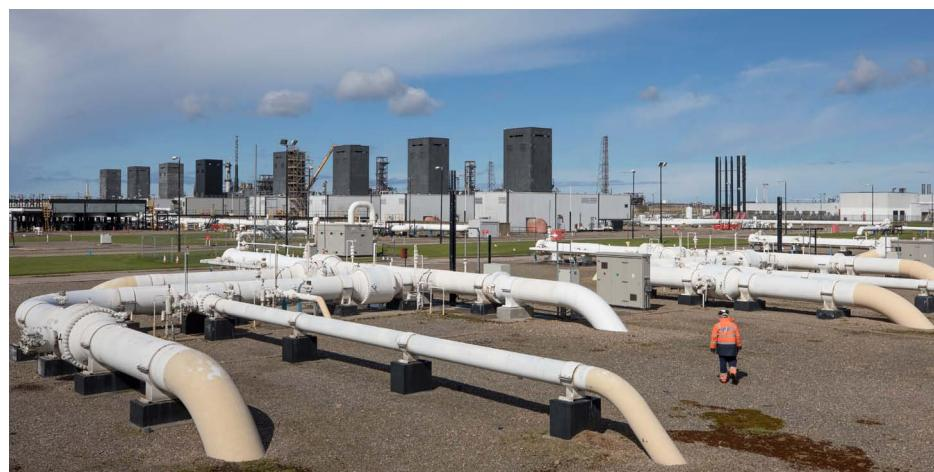
Pipelines are accurately asset managed through, amongst other activities, in-line inspection i.e. inserting a device within the pipeline. Currently we in-line inspect over 7,000 kilometres (99.5%) of our National Transmission System (NTS) using PIGs. However, PIGs are not suitable for pipework on AGIs and some other pipeline sections, for a number of reasons including, most notably:
