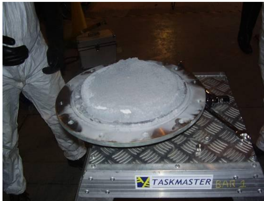
Figure 5.1 A – Example of SF 6 Contamination
