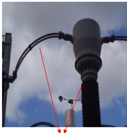
Figure 7.2A - Example of proximity of lower level equipment - Safety Distance to be maintained when applying portable Earthing Device(s) will be from the bottom of the CT housing not the conductor as indicated by the red arrows.
