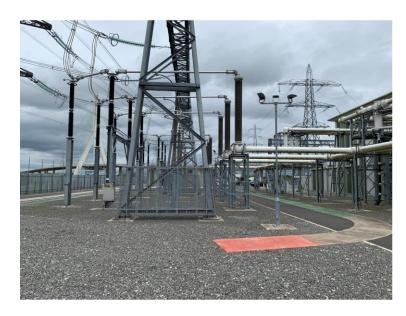
Photo 3. Illustrative view of the Substation showing GIB & AIS equipment connecting to a Gantry and OHL.
