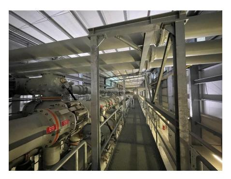
Photo 2. Illustrative view of the Substation GIS Hall taken at Connah's Quay.
