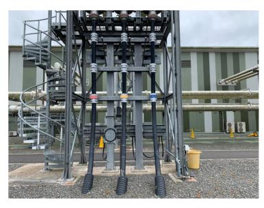
Photo 1. Illustrative view of the Substation taken at Connah's Quay showing outside of a GIS Hall & HVAC equipment.
