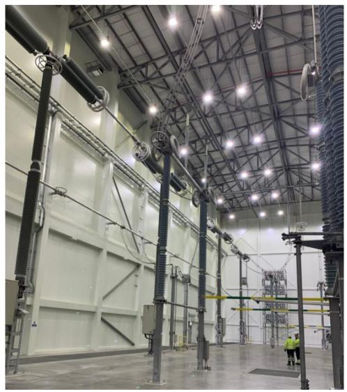
electrical clearances required at an operating voltage of 525kV. The photograph below shows a typical DC hall:
