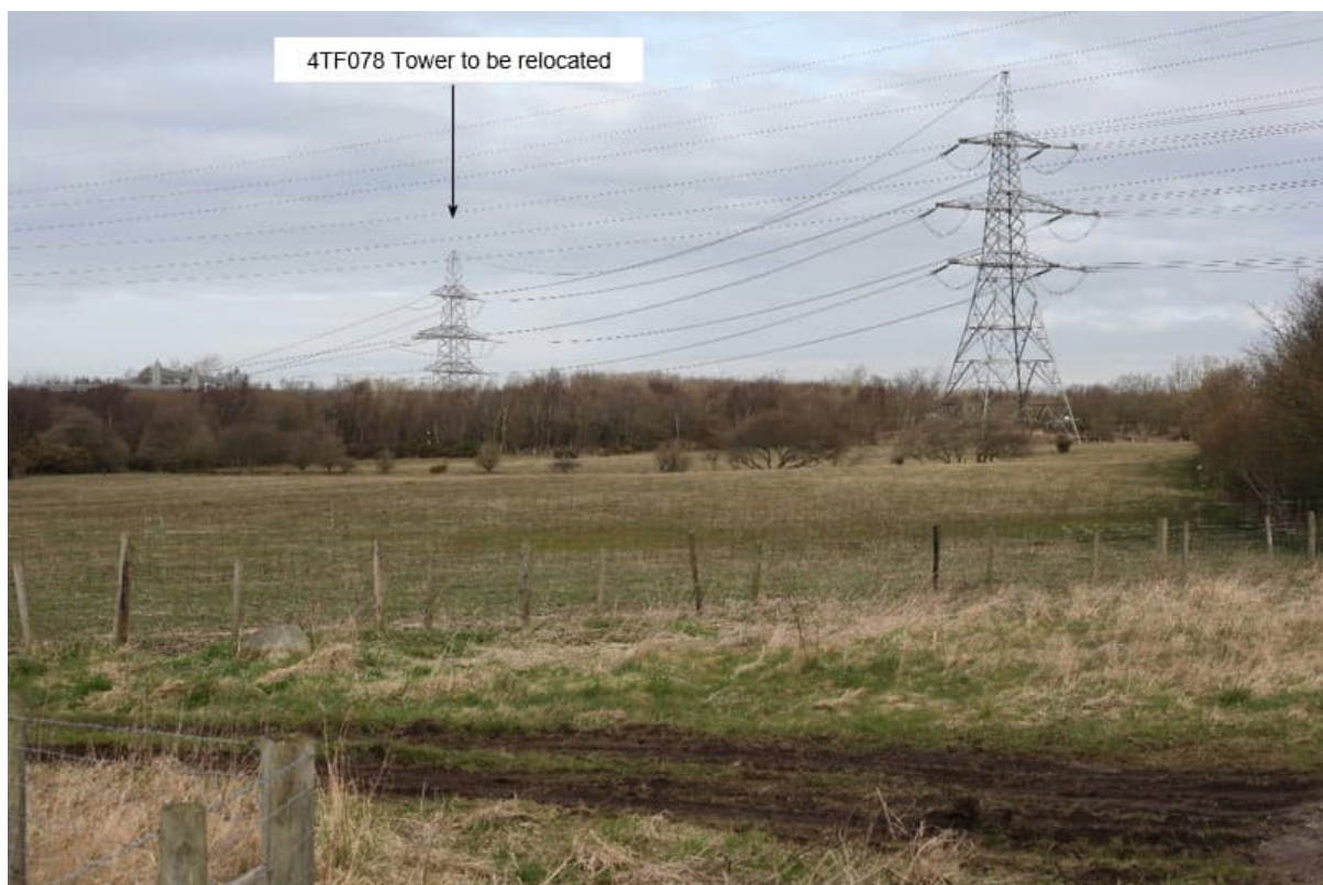
Figure 3-2 Image showing the visual effect following the removal of towers 4TF080 and 4TF079 and the relocation of 4TF078
