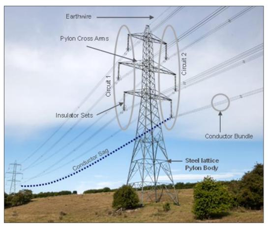
Figure 2-1 – Components of a Typical Transmission Connection
