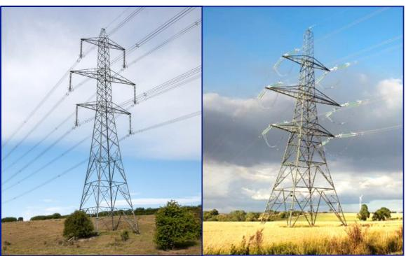
Figure 2-2 – Suspension Pylon (Left) and Angle Pylon (Right)
