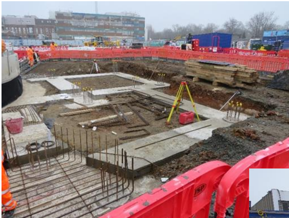
Headhouse foundations on the south side of the shaft
