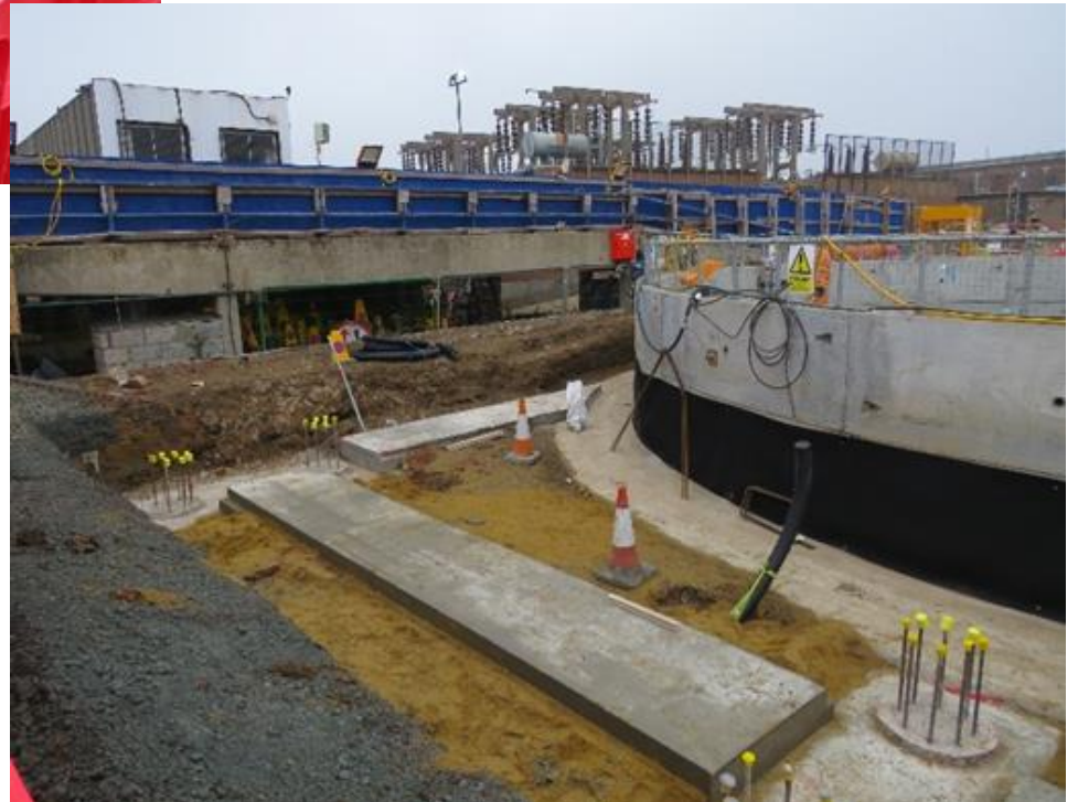
Headhouse foundations on the west side of the shaft
