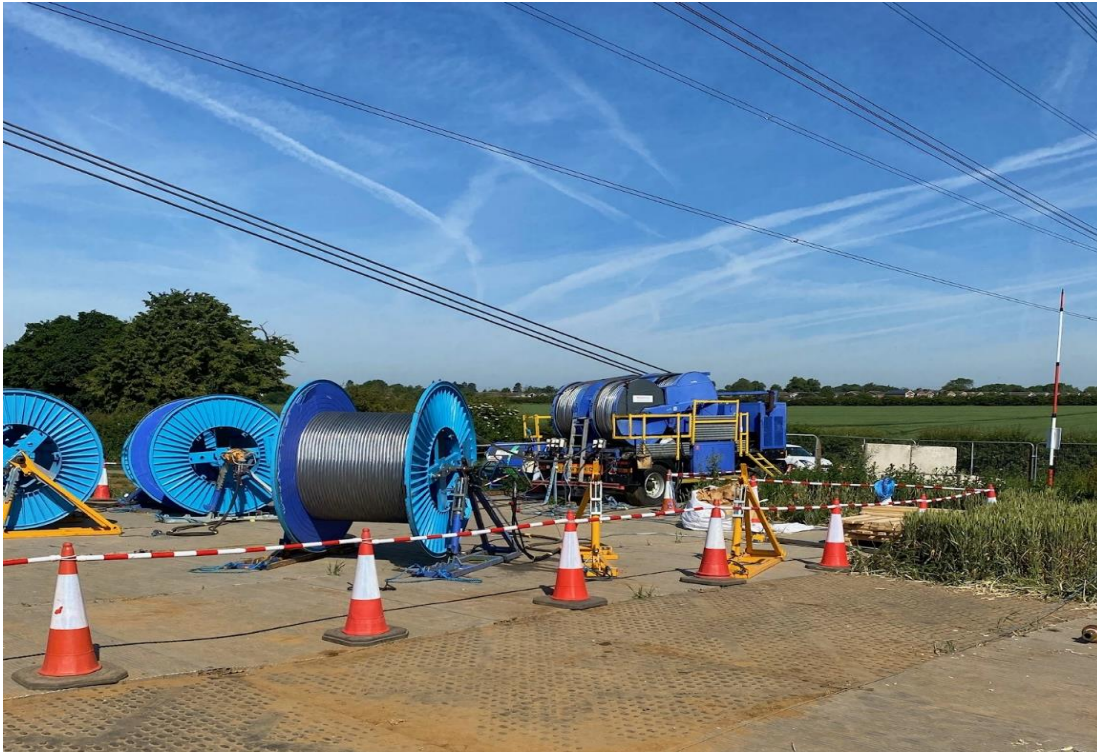
Layout of an Equipotential Zone (Ensure Positioned to Maximise Clearance to Adjacent Live Circuit)
