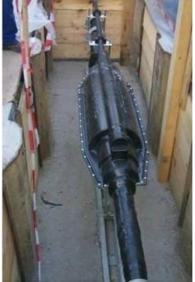
4.1 **Figure C.4: Cable Cross-Section and Joint**
