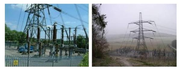
Figure C.5: Cable Sealing End Compounds
