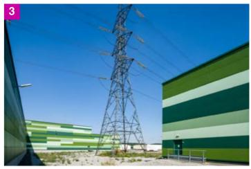
Development has been effectively planned around the transmission line. The pylon is accommodated with sufficient space provided for maintenance access.
