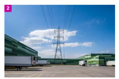
The design and arrangement of the development results in the effective utilisation of land beneath the transmission line. In places the space provides for loading and vehicular circulation while buildings occupy other parts with building heights adjusted accordingly.
