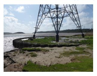
Pylon 4ZC030R foundations and cofferdam at the edge of the estuary channel
