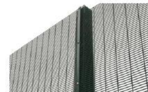
F Low level security mesh to base of south elevation
