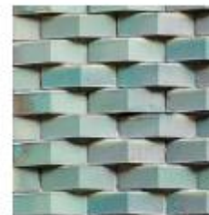
B 'Saw tooth' (angled) brickwork bands
