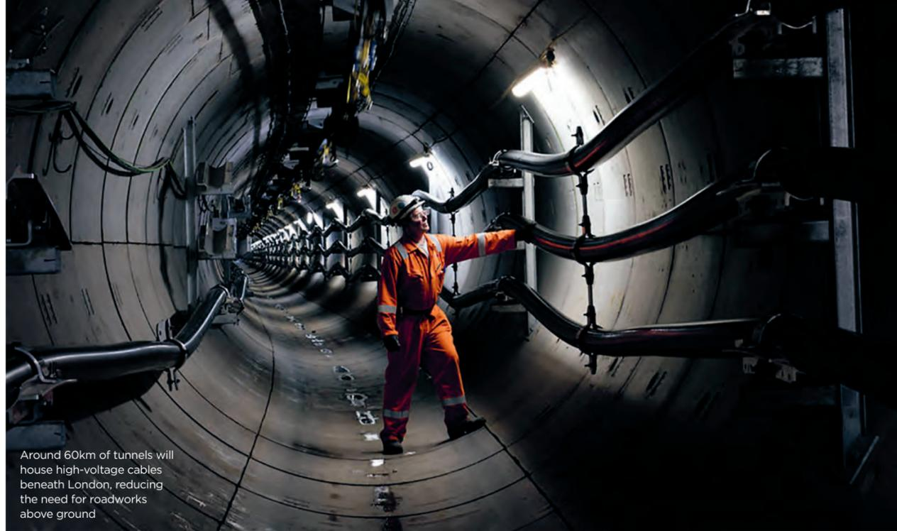
Around 60km of tunnels will house high-voltage cables beneath London, reducing the need for roadworks above ground
