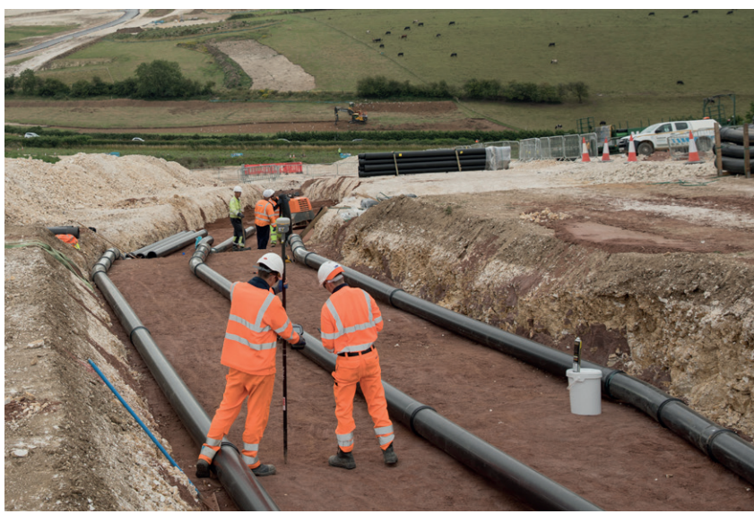
Cables will be installed 1-1.5 metres underground, as seen in the above image.
