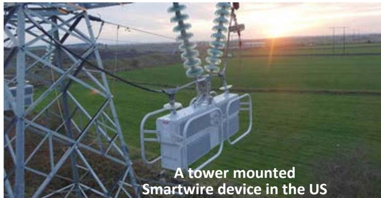
Figure 5 – Smartwire Device Installed on Overhead Line
