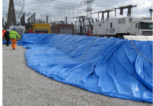
Figure 10.3 Example removable flood barrier use
