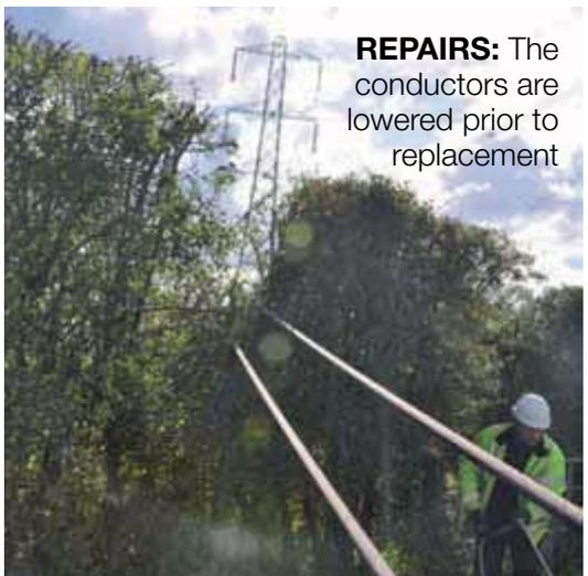
**REPAIRS:** The conductors are lowered prior to replacement
