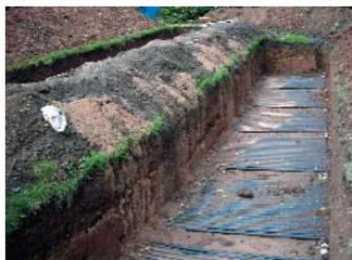
Pipework is laid in the ground to pick up the heat for the ground source heat pump
