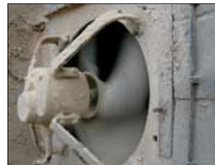
Dirty fans and guards reduce the efficiency of ventilation systems by as much as 60 per cent
