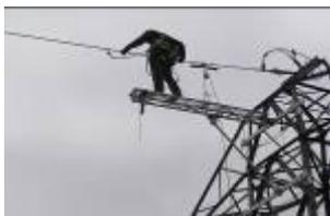
**Earthwire Platform** – this platform is being developed to provide a suitable access/egress platform whilst carrying out maintenance on earthwires. The initial prototype has been trialled, identifying a change to the specification and design parameters. The second prototype has been manufactured and tested. Field trials are to be completed to ascertain the suitability of the current design and any required design changes.
