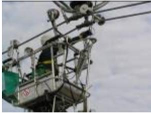
**Trolley Jump Kit** – the aim is to develop a lightweight jump kit which will be used to allow suspension insulators to be passed within the overhead line conductor trolleys. First prototypes of new jump kit have been trialed and a number of improvements identified. A second prototype has now been manufactured and tested. Field trials are now required to ensure the new equipment works efficiently and to identify any further modifications.
