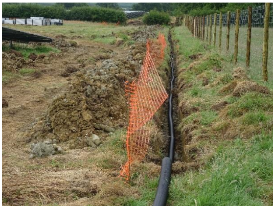
Photos 8 and 9: Cable Installation
