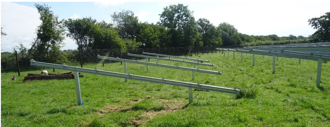
Photos 5 and 6: Constructing the Frame
