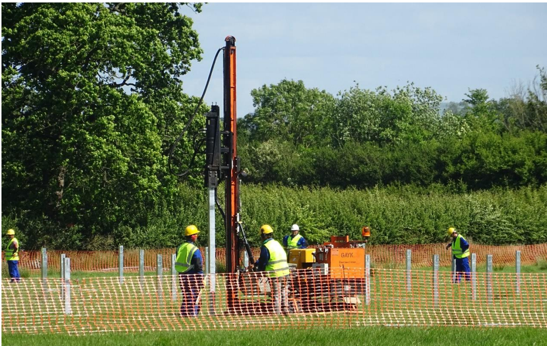
Photo 2: Inserting a Stanchion
