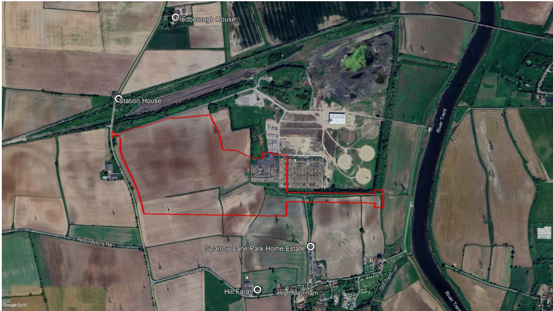
Figure 1.3 Aerial view of Scheme red line boundary and identified NSRs – Source © Google Earth
