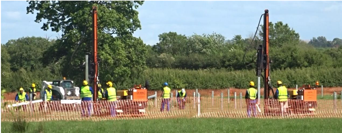
Photo 3: Team Installing Panels
