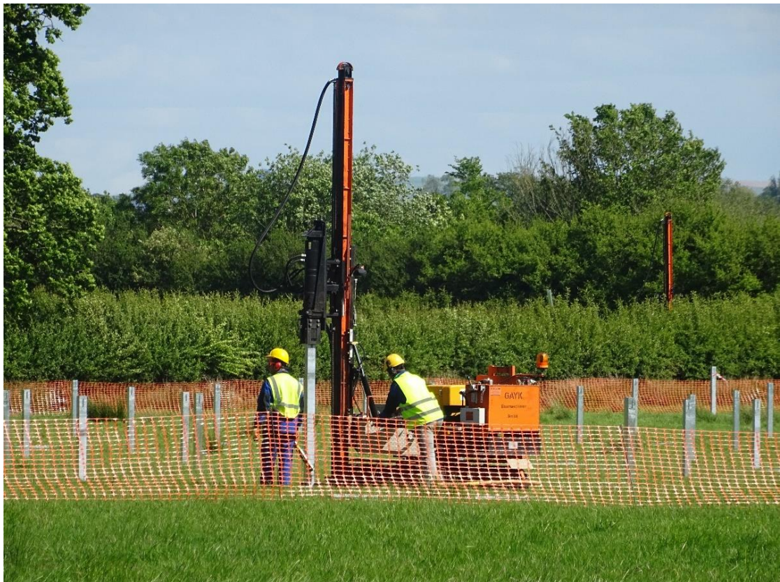
Photo 1: Post Rammers at Installation Stage
