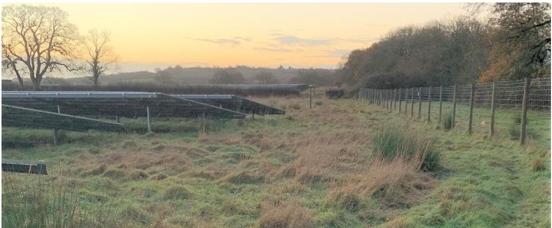
Photo 11: Panels After Five Years
